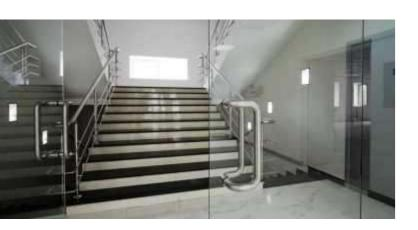
Glass doors are available for houses, offices, malls and all types of spaces. Doors can be bolt, motor, sliding, and photocell (radar). Depending on the purpose and size, tempered glass used can be 8 mm or 10 mm thick Profiles and accessories are produced in Germany, Denmark and Turkey.
